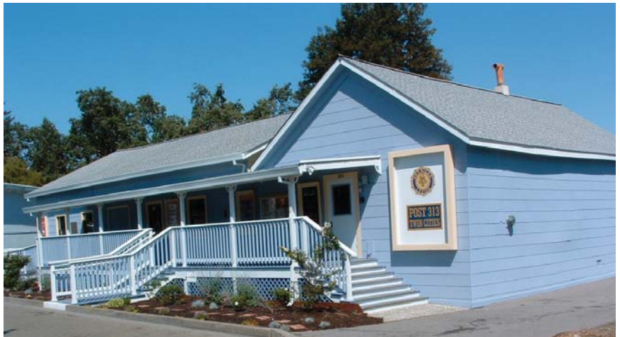
August Improvements to Driveway Side of Post
